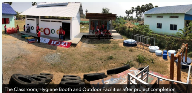
The Classroom, Hygiene Booth and Outdoor Facilities after project completion
